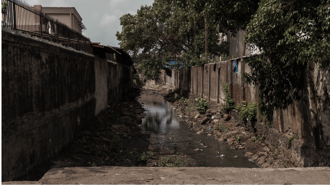
Pipeline, The MIDC Industrial Park in Mumbai, India. Personal photograph by author. June 15, 2019.
